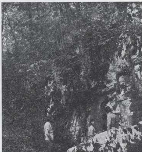
Sl. 30 Rožanec — pri konservatorskih delih Fig. 30 Rožanec — during the conservation works
