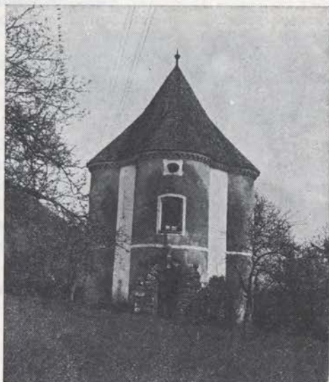
Sl. 36 Soteska — vrtni paviljon po obnovi l. 1975 Fig. 36 Soteska — the garden pavilion after its renewal in 1975
